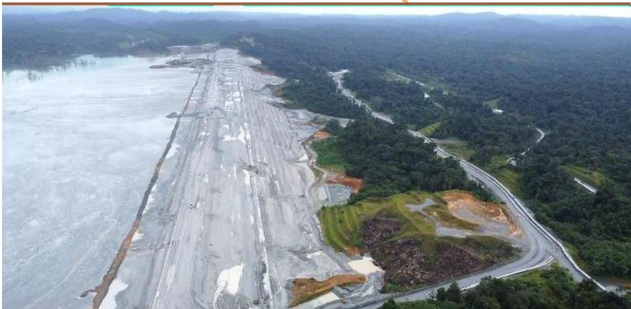
Figura No. 20, IMR muro Norte
