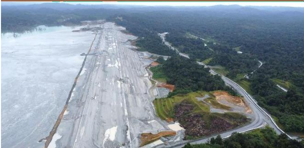
Figura No. 17, IMR muro Norte
