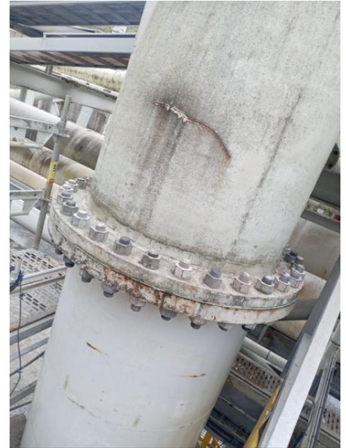
Gasket replaced
